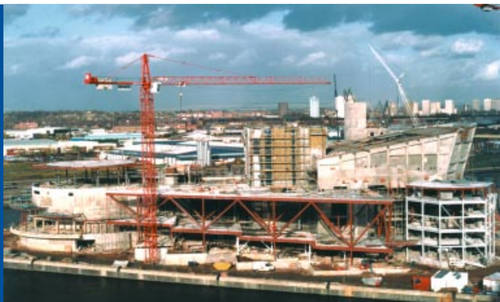
Well Under Way - The Lowry construction site on Salford Quays
